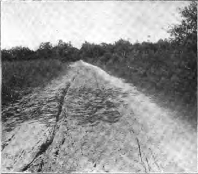
New Gretna road, Burlington Co., before improvement.
